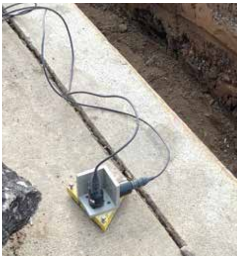
Figure 4. Continuous monitoring of vibrations adjacent to a shallow excavation.
