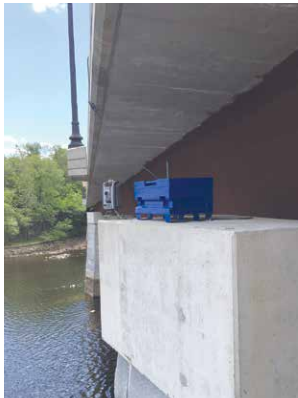
Figure 8. Automated system for the survey of a bridge.
